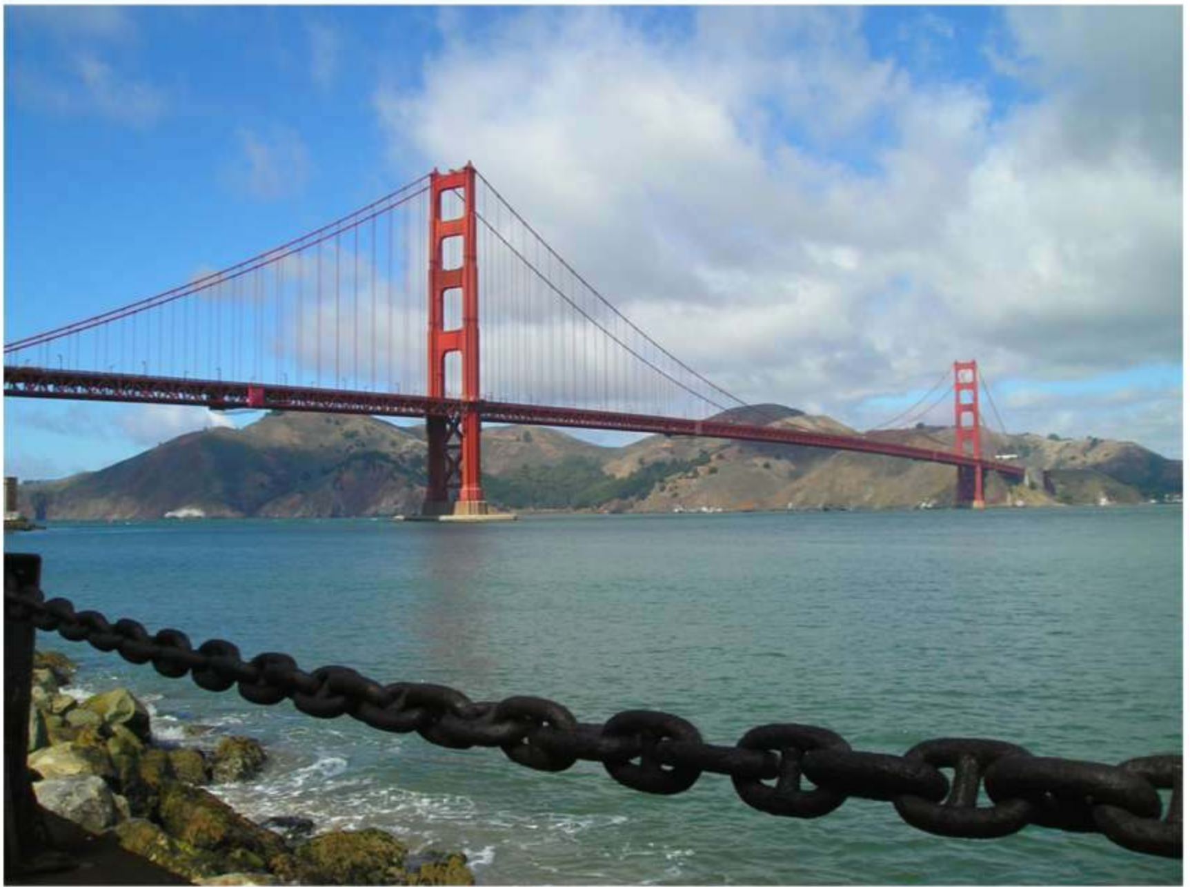
Golden Gate bridge, San Francisco
