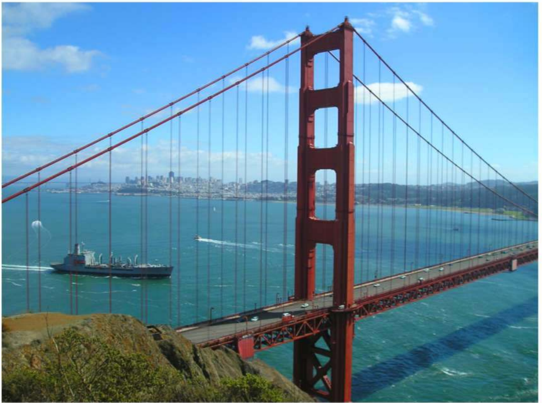
Golden Gate bridge, San Francisco
